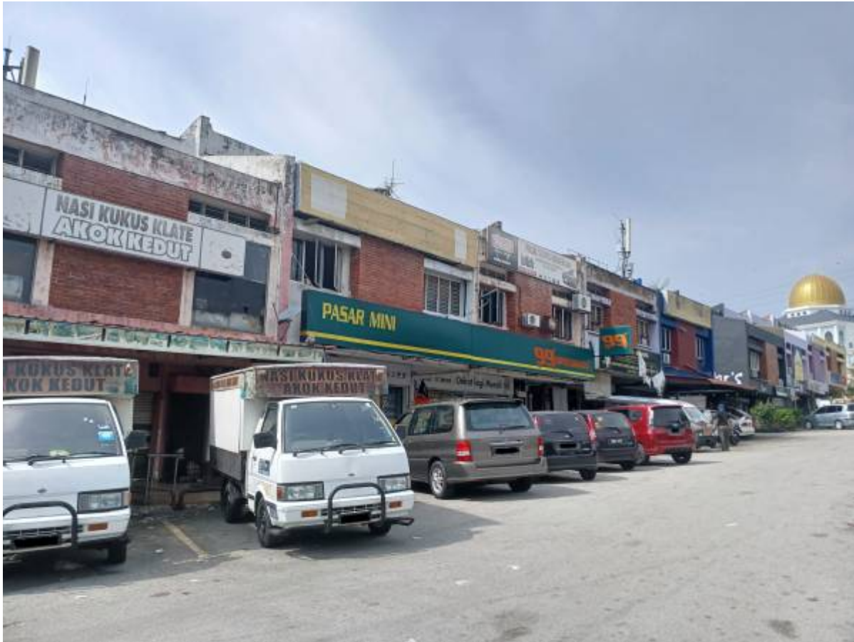
No. 4, Jalan 1/4 (99 Speedmart) (Gambar: Sazli Shahrir, 2025).
