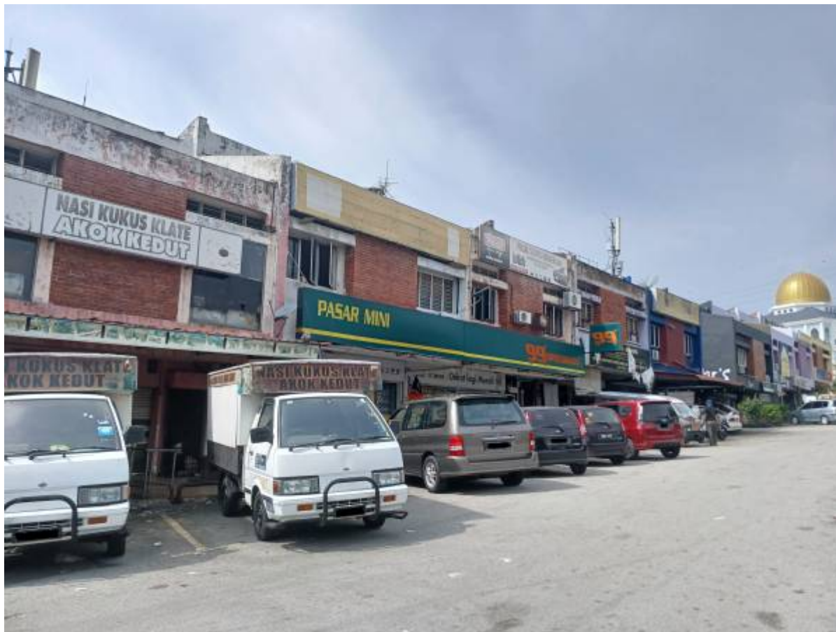
No. 4, Jalan 1/4 (99 Speedmart) (Gambar: Sazli Shahrir, 2025).
