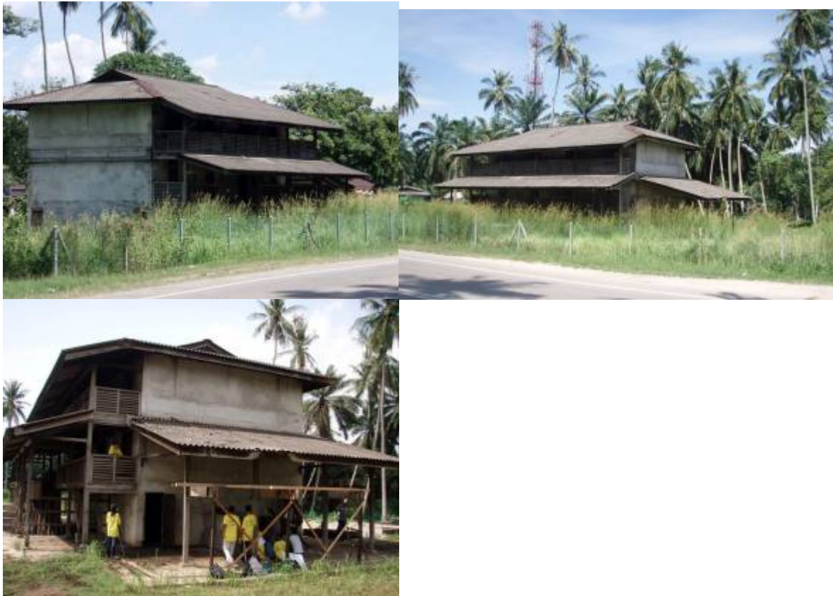
Sebelum dibaikpulih. Kiri: "Blackened, abandoned, dilapidated and ignored (2006)" . Tengah: "The rubber smokehouse before restoration" . Kanan: "Children learning how to conduct a dilapidation survey (2006)"
