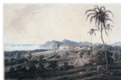
Glugor House, Penang
