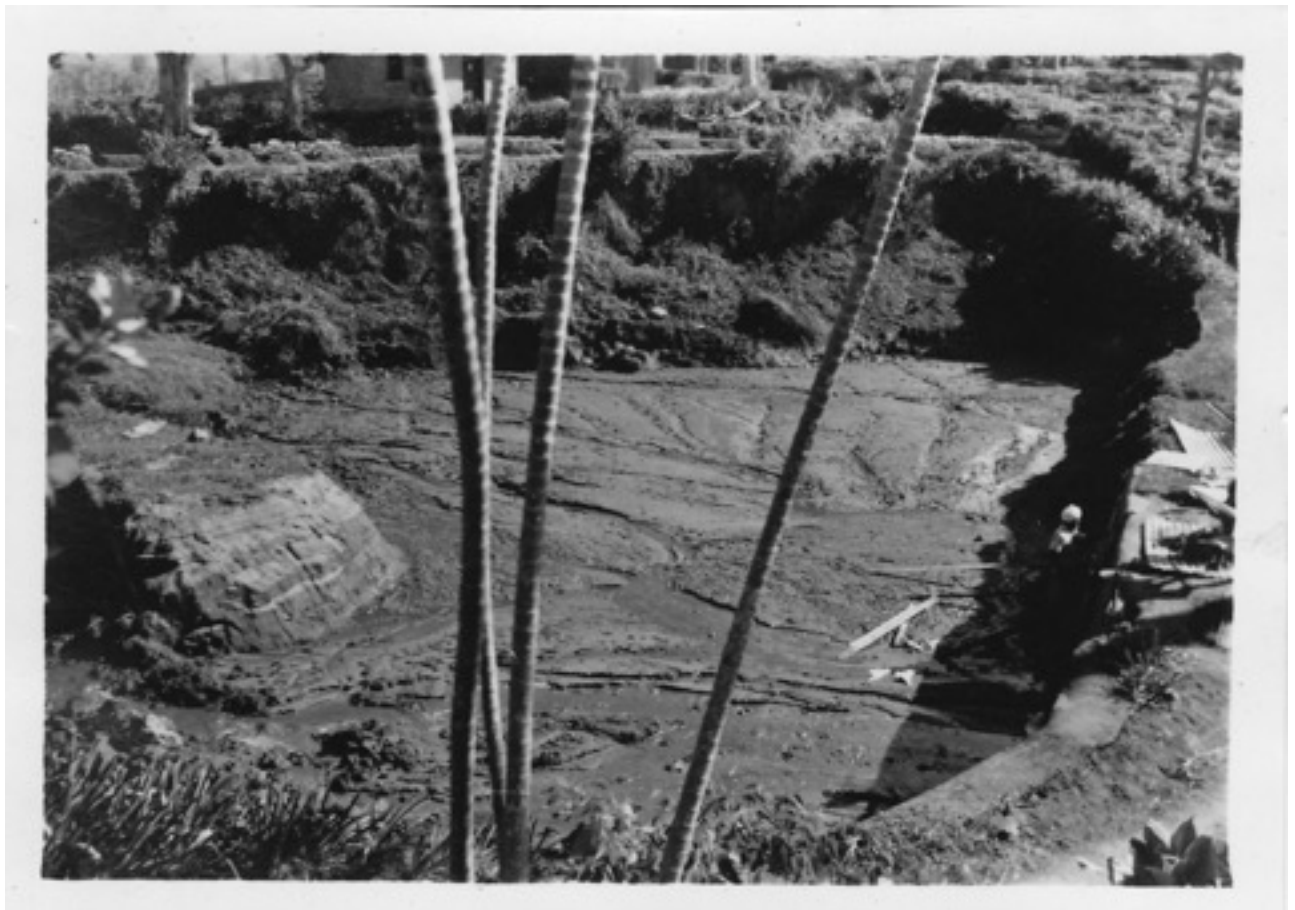
The disused dam in the process of being de-silted. The sluice is in the middle at the right.
