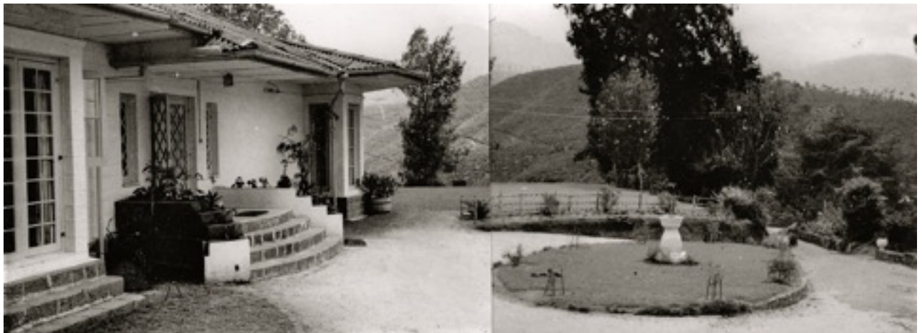
Alton Managers' bungalow c.1964. Redesign of forecourt in progress.
