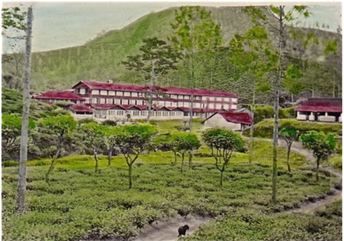
Glenlyon factory (rear) - 1952.
