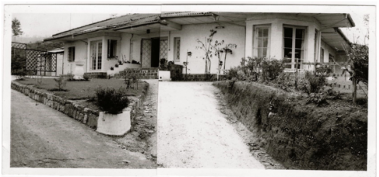
Alton Managers' bungalow c.1964. Redesign of forecourt in progress.
