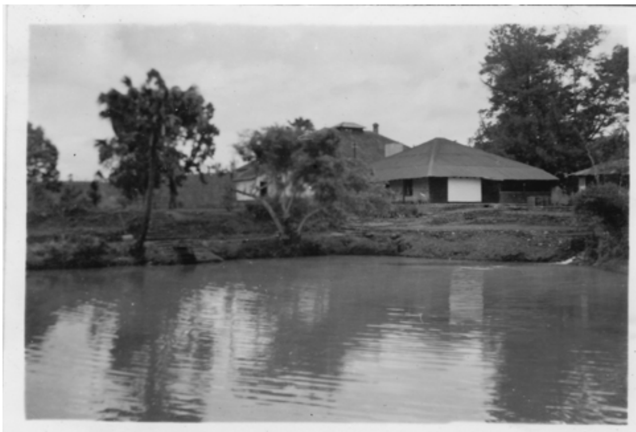
The refilled dam with the rear of the bungalow in the background.
